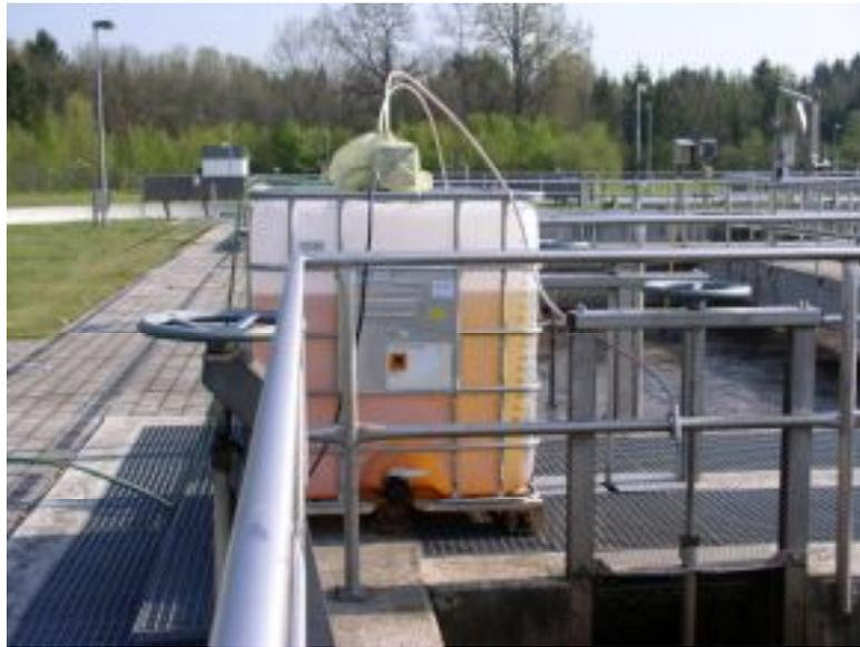
**Figure 3: Dosing system for stabilized folic acid (sewage treatment plant in Bavaria an der Isar)**
